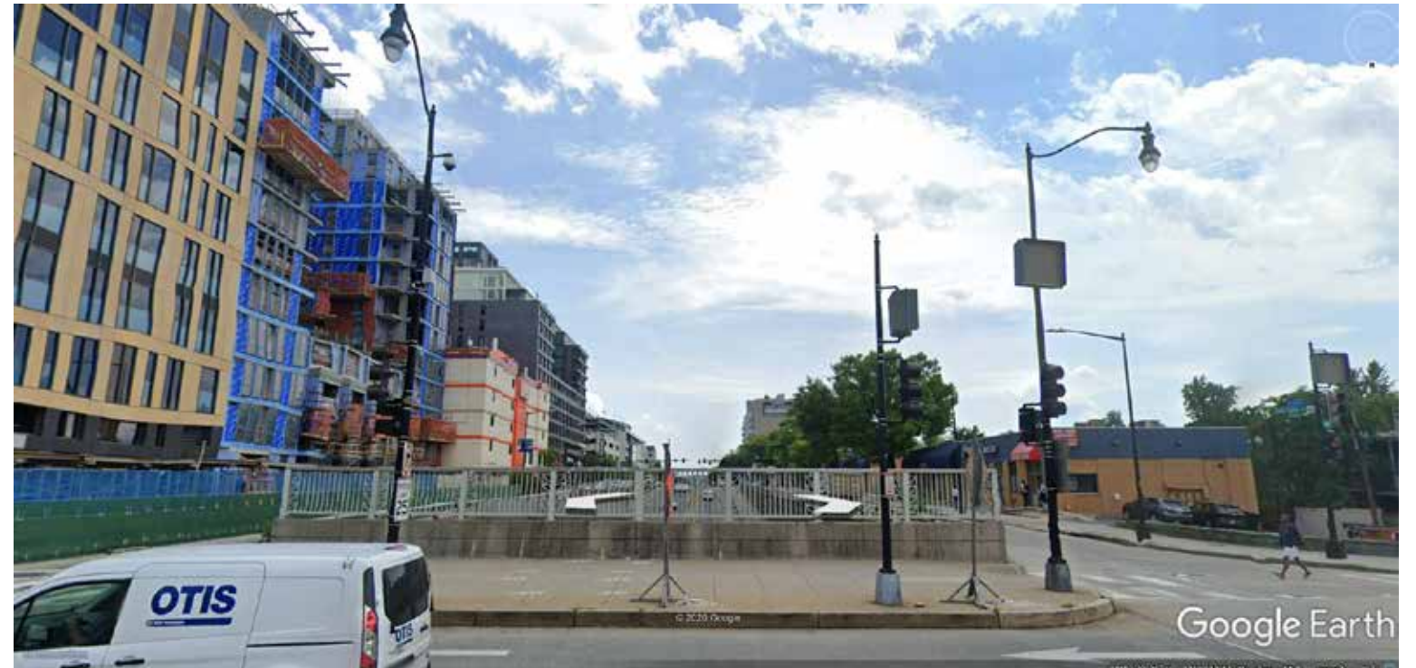
LOOKING NORTH TO BRIDGE
